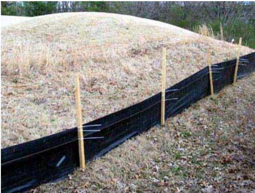
Properly Installed Silt Fence
