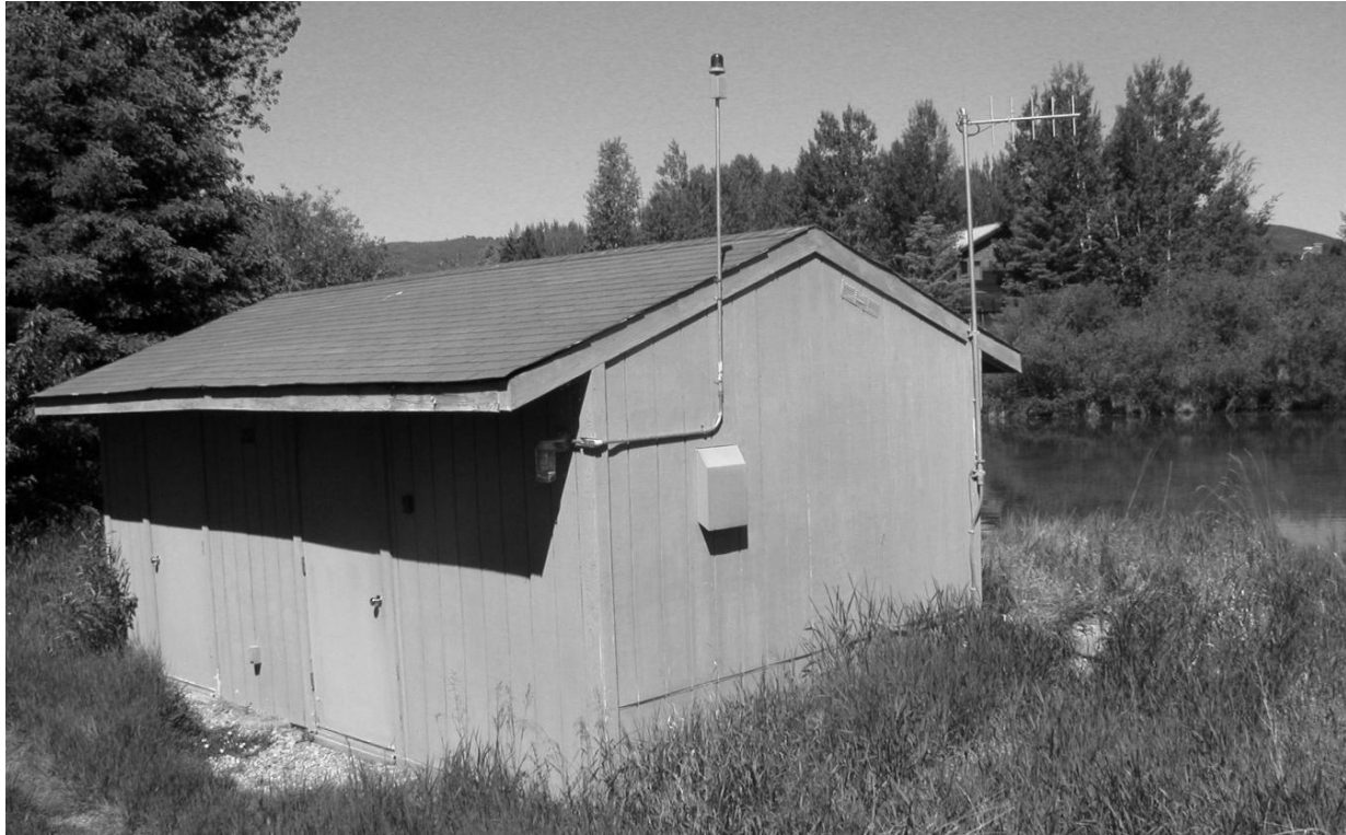
Drinking water treatment building. Note the warning light and telemetry antenna on the building and the third augmentation pond in the background.
